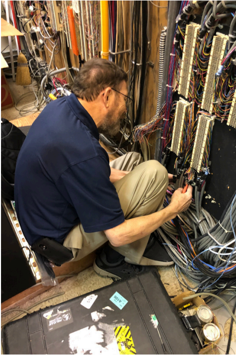
IRC's Howard Jorenby preparing wires for the installation of the IRC VSCU-1000 voting system
